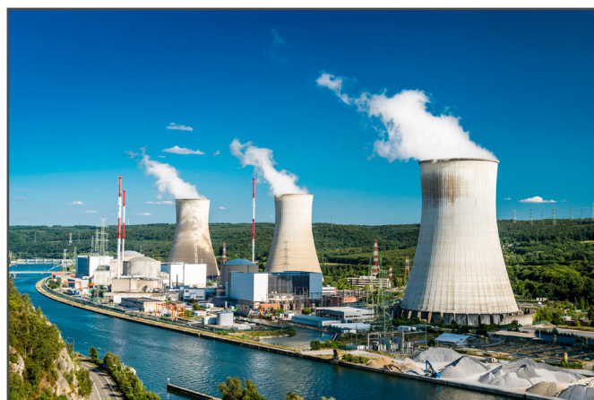
Cooling water control for power plants
